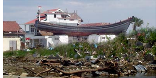
Runup can often be inferred from the vertical extent of dead vegetation, from debris normally found at ground level that are observed stuck on electric wires, in trees, or at other heights, and from water line marks left on building walls. In extreme cases, cars, boats, and other heavy objects have been lifted and deposited atop buildings. Banda Aceh, Indonesia, 26 December 2004. Photo courtesy of C. Courtney, Tetra Tech EMI.
