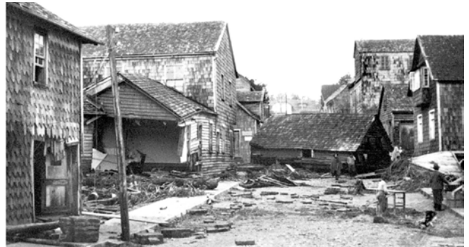
Damaged caused by the 22 May 1960 Chilean tsunami. Photo courtesy of Ilustre Municipalidad de Maulin, USGS Circular 1187.
