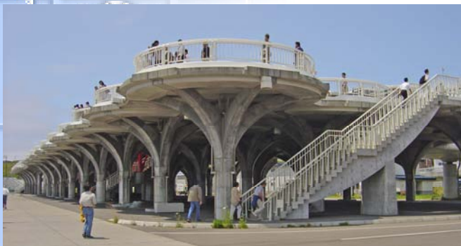
Elevated platform used for tsunami evacuation that also serves as a high-elevation scenic vista point for tourist. Okushiri Island, Japan. Photo courtesy of ITIC.
