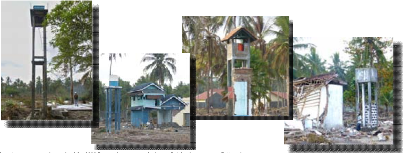
Water towers commonly survived the 2006 Pangandaran tsunami where adjoining houses were flattened.
