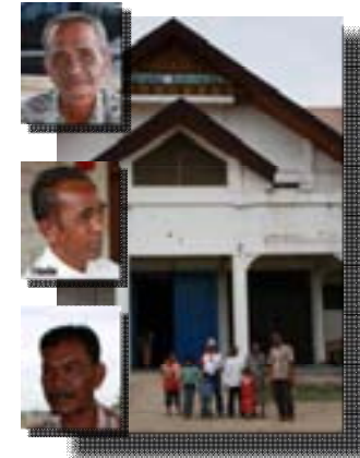
The photograph above shows the Serambi Indonesia Daily building. Fifty-two people survived by escaping to the second floor of this building. Among them were Mochtar, Ibrahim, Hasbi and Rohani (back row, right to left) and Rohani's children, Intan, Muhajirin and Magdalena (front, right to left).
