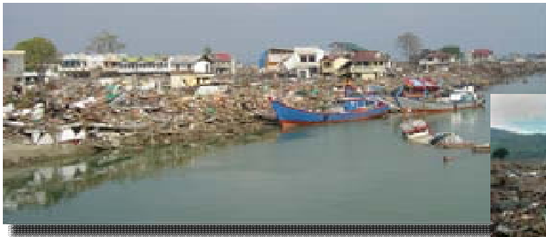
Several two-storey buildings withstood the 2004 Aceh tsunami even though they were close to rivers.
