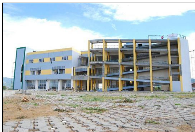
Figure 10. Tsunami Disaster Management and Research Center Building, Syiah Kuala University, NAD (TDRMC Unsyiah, 2008)
