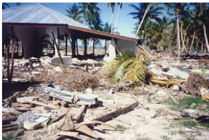
Damage to infrastructure (Biak, 1996)
