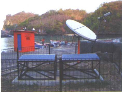
Figure 19. Tide Gauge Station Sadeng
