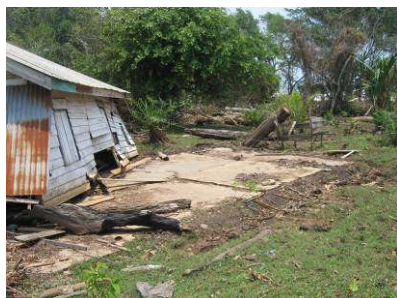
The house was moved from its original location due to the tsunami hydraulic force in Muko muko, Bengkulu
